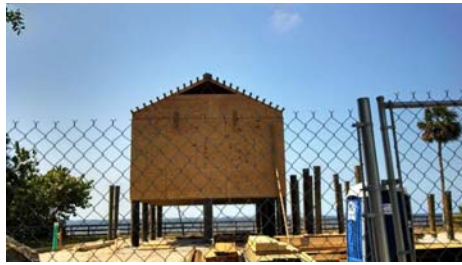
New Bathroom Facility Under Construction
