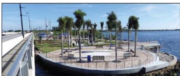
A new seawall is just one aspect of the Harbor Walk project, which eventually will connect the east side of the northbound U.S. 41 bridge to Bayshore Live Oak Park on the west side.
